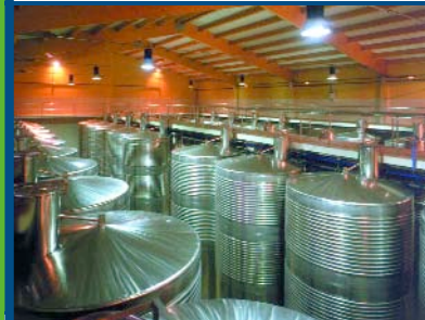
Winery wastewater treatment plant Spain
