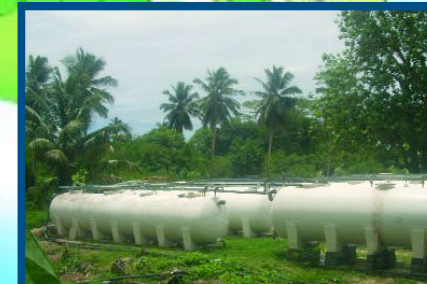
WWTP - 300 m 3 /d logistic yard Nigeria
